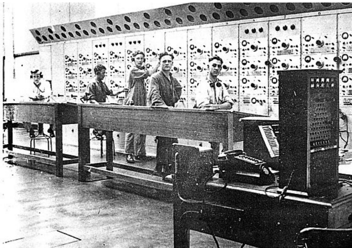
Fig. 38: Kingsley HF Radio Receivers, Type AR7 – WW2 RAAF Remote Receiver Station at Werribee. Source: Butler, Lloyd VK5BR. ( http://www.qsl.net/vk5br/AR7.htm ).
